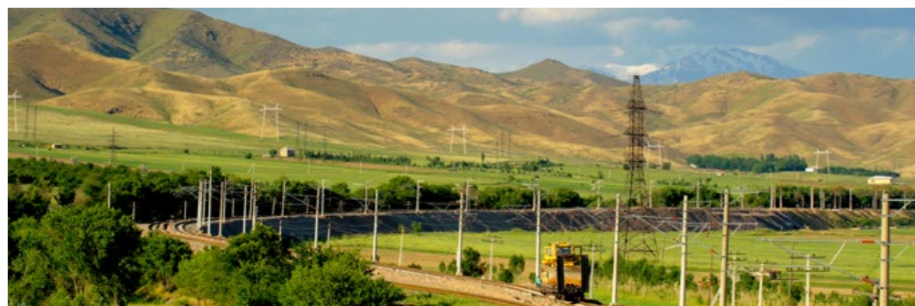
The Uzbekistan Railway Electrification Project
