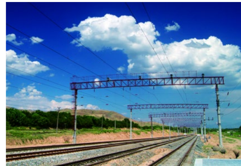
The Uzbekistan Railway Electrification Project site
