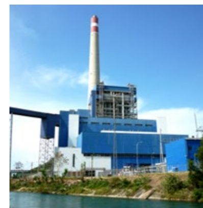
Suralaya 1x625MW Coal-fired Power Plant Project in Indonesia
