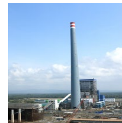
Adipala 1x660MW Supercritical Coal-fired Power Plant Project in Indonesia
