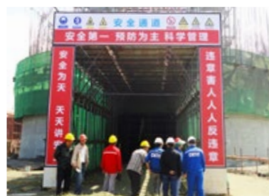
Emergency Access for the chimney construction at the Adipala Power Plant Project
