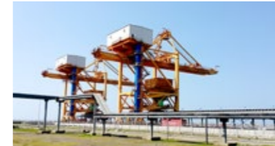
Adipala Power Plant Project
