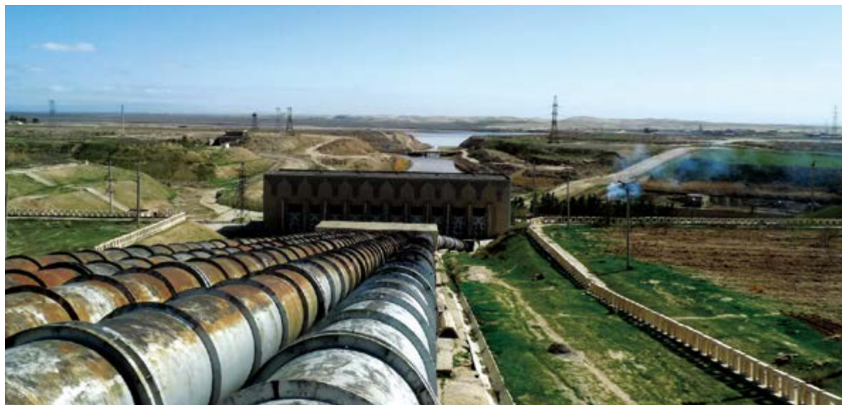
乌兹别克斯坦阿姆布哈拉 1 号新建泵站 The New Amu-Bukhara I Pump Station in Uzbekistan
