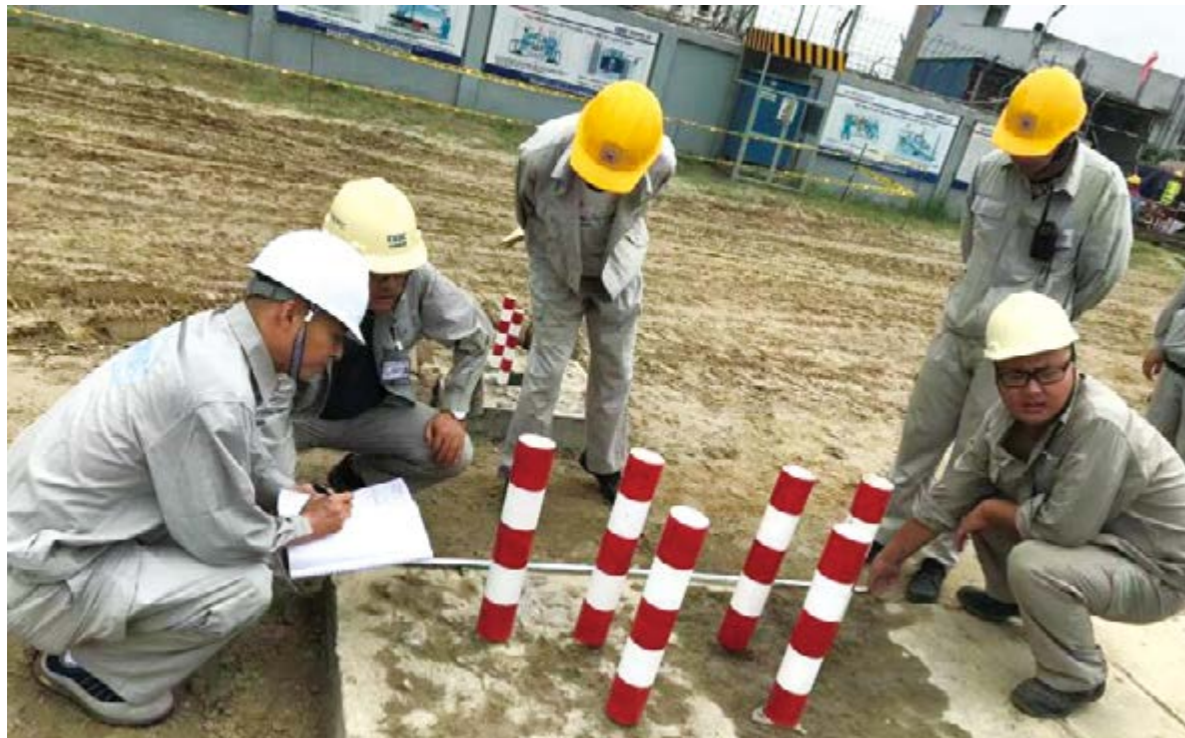
阿苏甘杰东燃机电站项目质量抽查实测 Spot measurement of the quality of the Ashuganj Power Plant (East) Project
