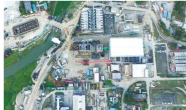
阿苏甘杰东 400MW 联合循环燃机电站项目 The Ashuganj 400MW Combined Cycle Power Plant (East) Project
