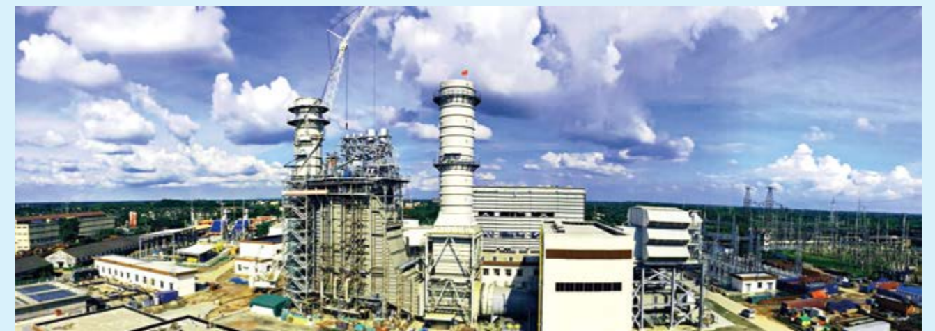
古拉绍燃机电站项目全景图 Panorama of the 365MW Combined-cycle Gas-turbine Power Station Project in Ghorasal, Bangladesh
