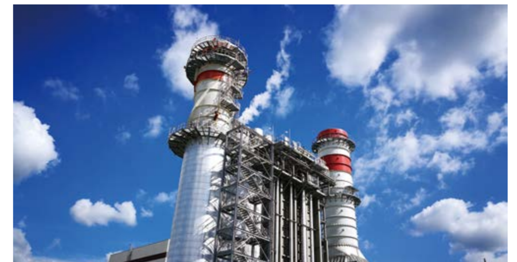
古拉绍燃机电站项目一角 A glimpse of the 365MW Combined-cycle Gas-turbine Power Station Project in Ghorasal, Bangladesh
