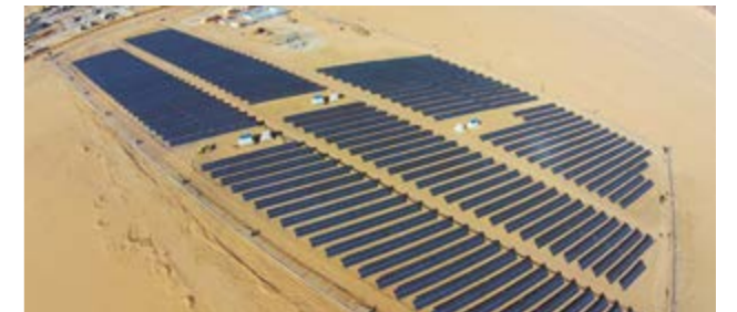
阿尔及利亚 25MW 光伏电站项目全景 The panorama of the 25MW Photovoltaic Power Station project, Algeria
