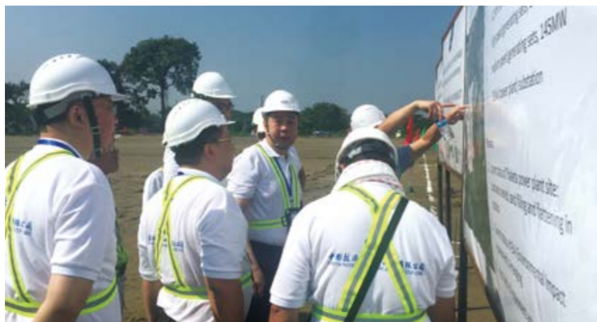
缅甸快速发电项目开展安全大检查 Safety inspection at the Fast Power Generation project in Myanmar
