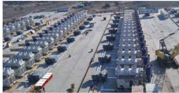
缅甸敏建 90MW 燃气电站项目顺利通过试运行 The 90MW Gas Powered Plant project in Myingyan, Myanmar passing trial operation
